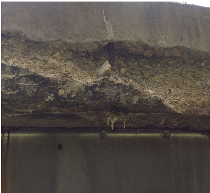
PHOTO 1 Description Right outside edge of deck spalled with 4" of exposed rebar.
