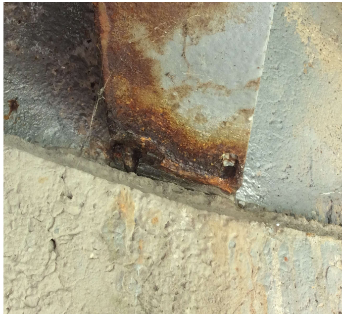
PHOTO 1 Description Bottom flange of Girder 11 at end of Span.
