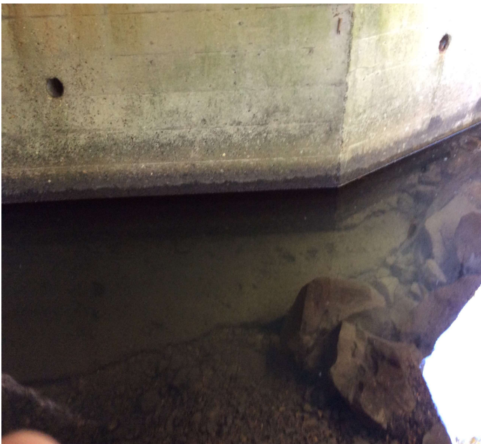
PHOTO 1 Description Footing @ Abutment 1 is exposed.
