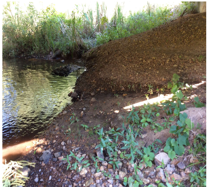
PHOTO 2 Description Channel has realigned to Abutment 1 with scour developing.
